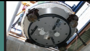
Proton therapy equipment is installed as construction of the Perelman Center nears completion.
